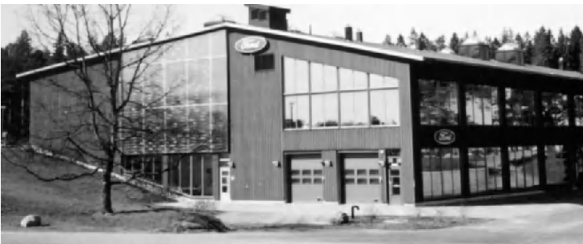
Fig. 4.1 South-facing façade of Greenzone Building 1.
