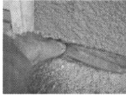
FIG. 5—“Tag and fix” approach to sealant testing.
