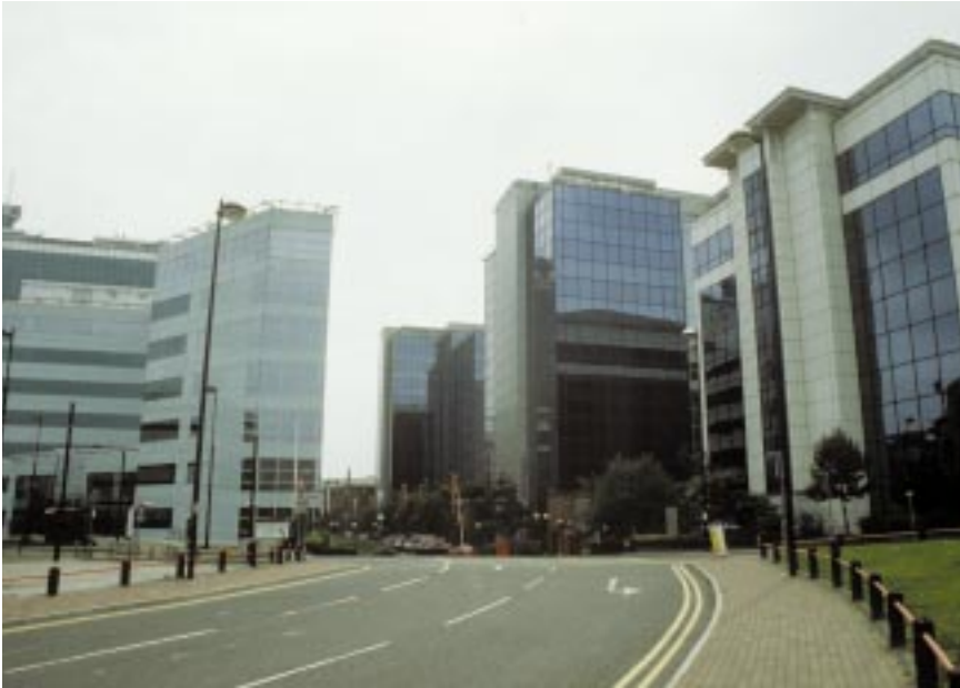
Figure 26: Exchange Quay – the approach to the scheme, high density, corporate and international in image
