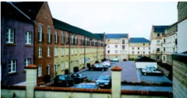
Car parking dominating space
