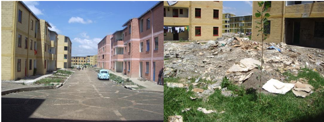
Linear arrangement of building verses building at right angle ( Photos of sample neighborhoods in Addis Ababa)
