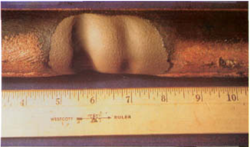
Figure 17.5 Utility superheater tube cut by steam leaking from an adjacent tube that failed at a manufacturing defect. Note the smoothly undulating surface and removal of red and black oxides and deposits in the wasted area.
