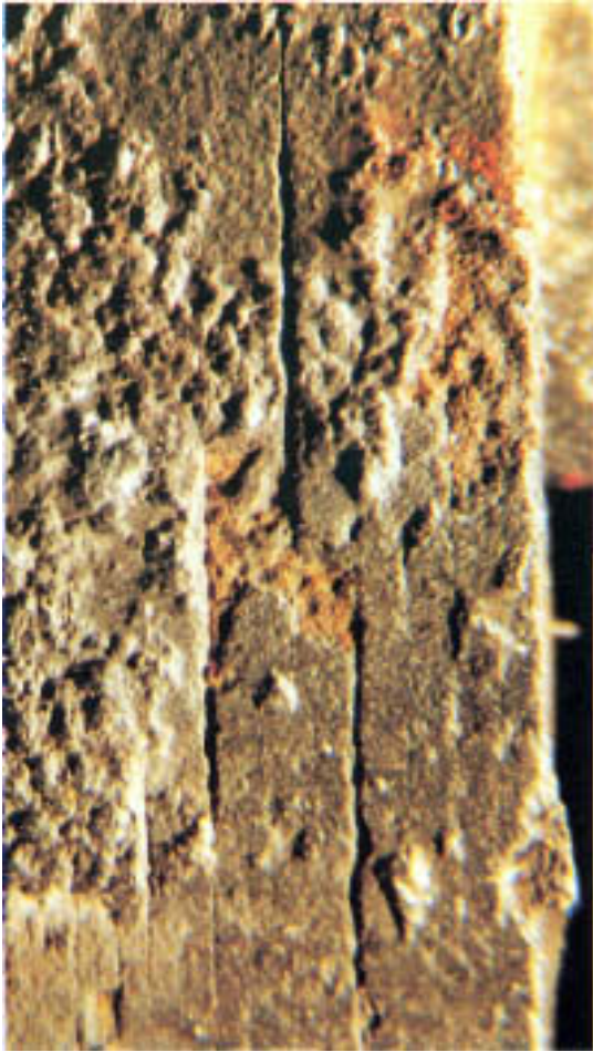
Figure 15.11 Secondary corrosion-fatigue cracks on external surface. (Magnification: 6.5X.)
