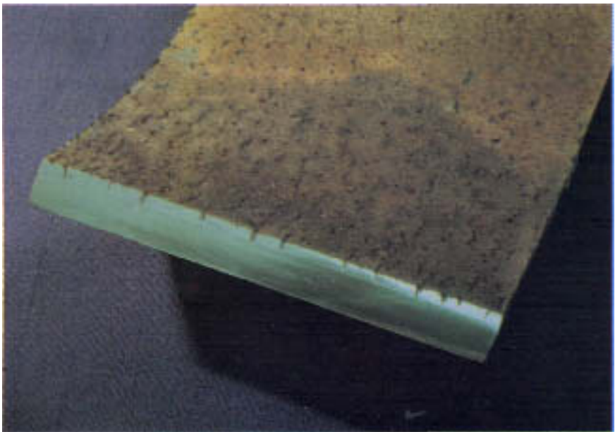
Figure 15.4 Transverse cracks originating on the internal surface.
