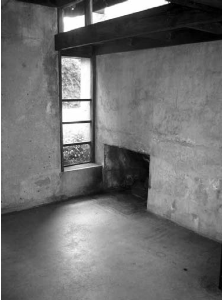
The interior in Rudolf M. Schindler's Kings Road House, Los Angeles, 1921–2.
