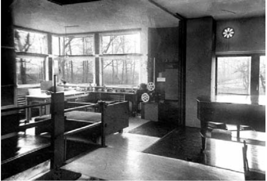
The first floor of the house designed by Gerrit Rietveld for Mrs Truus-Schroeder, Utrecht, 1924.
