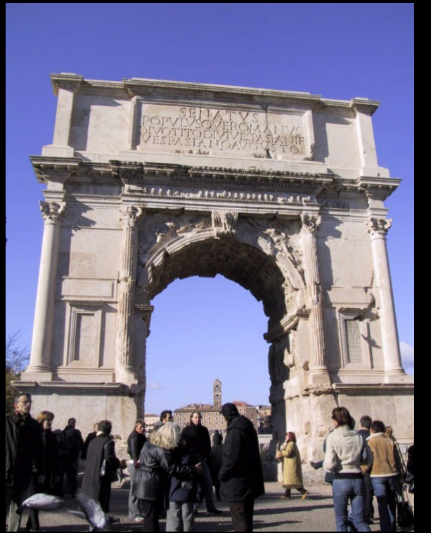
Arch of Titus 81 CE, marble over concrete core, 50' high x 40' wide, Rome, Italy
