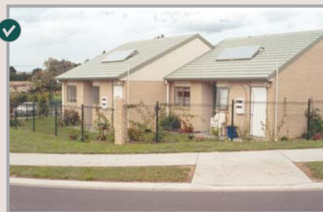
HNZC housing with supplementary solar water heating.
