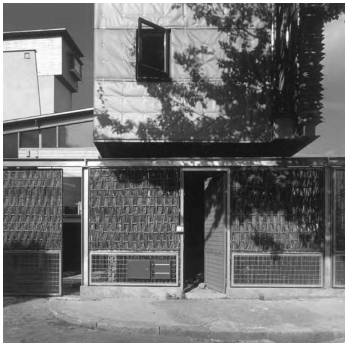
Sarah Wigglesworth and Jeremy Till, Wattle/steel fence (2000), Stock Orchard Street. Photograph: Paul Smoothy (2001).
