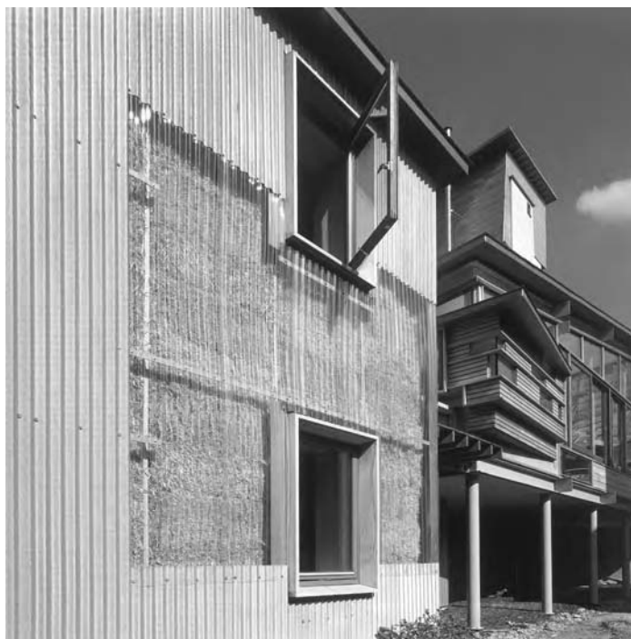
Sarah Wigglesworth and Jeremy Till, Straw walls (2000), Stock Orchard Street. Photograph: Paul Smoothy (2001).
