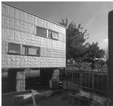
Sarah Wigglesworth and Jeremy Till, Quilted rainscreen to the office (2000), Stock Orchard Street. Photograph: Paul Smoothy (2001).
