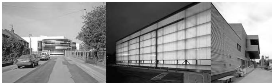
The Gateway 'parts' – the 'peanut', academy hall and stand: Fluid (2004). Photographs: Hélène Binet and Kim Trogal (2004) (Fluid).
