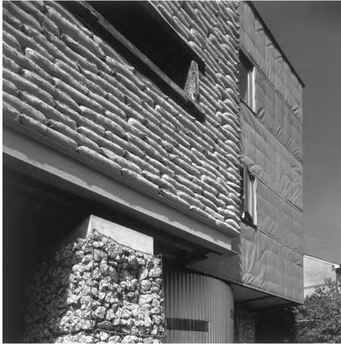
Sarah Wigglesworth and Jeremy Till, Sandbag wall (2000), Stock Orchard Street. Photograph: Paul Smoothy (2001).
