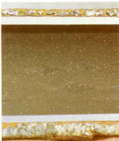
Figure 1.15 Sparkling black magnetite crystals on internal surface of a wall tube. Crystals are formed by precipitation on surfaces, or are transported from preboiler areas.
