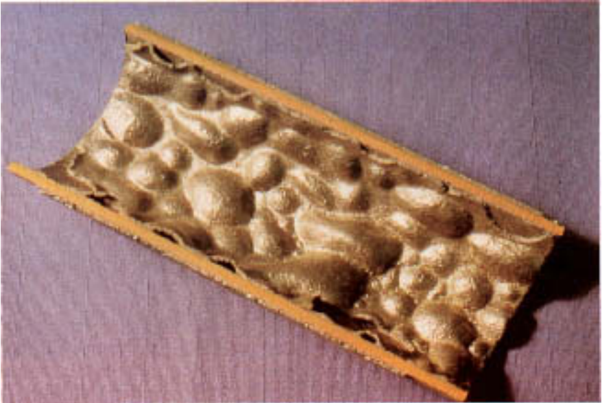
Figure 2.4 Thick, blistered magnetite layer on internal surface of 150-psi (1.0-MPa) tube. Oxide was formed during dry firing of boiler. Metal temperatures approached 2000°F (1100°C), causing slow, “viscous” flow of magnetite.
