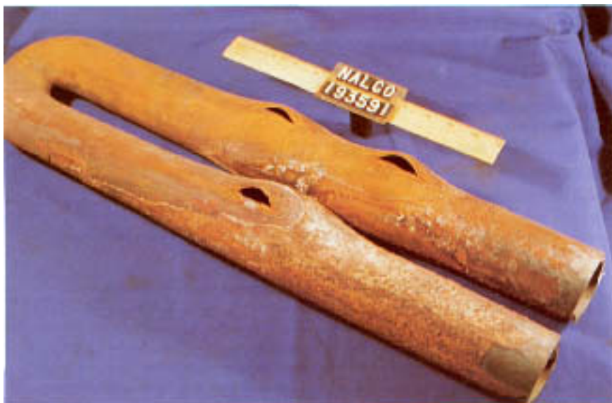
Figure 2.13 Bulged and ruptured superheater U-bend. The legs are slightly expanded.
