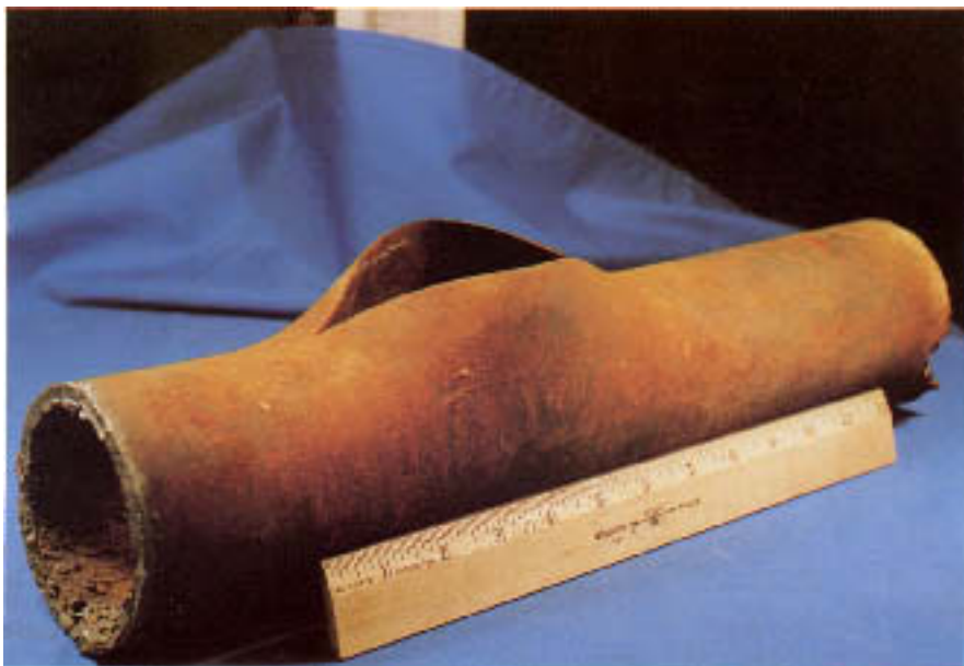
Figure 3.4 A rupture at a single bulge. The tube had experienced long-term overheating, followed by a brief episode of severe overheating.
