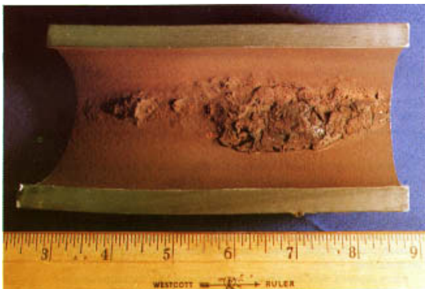
Figure 4.7 Patch of hard iron oxides on internal surface.
