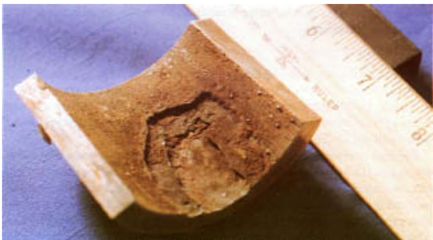
Figure 4.6 Region of caustic gouging along internal surface.
