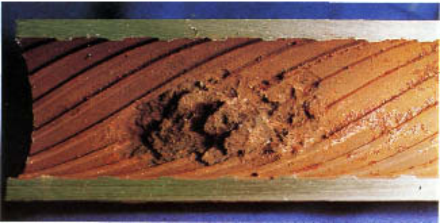
Figure 4.9 Thick, irregular mound of hard iron oxides covering perforation.
