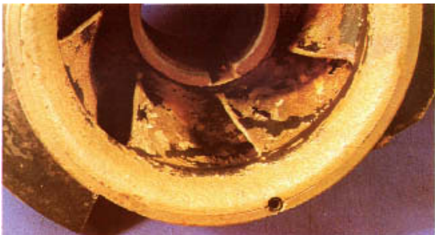
Figure 5.5 Chelant corrosion on feedwater pump.
