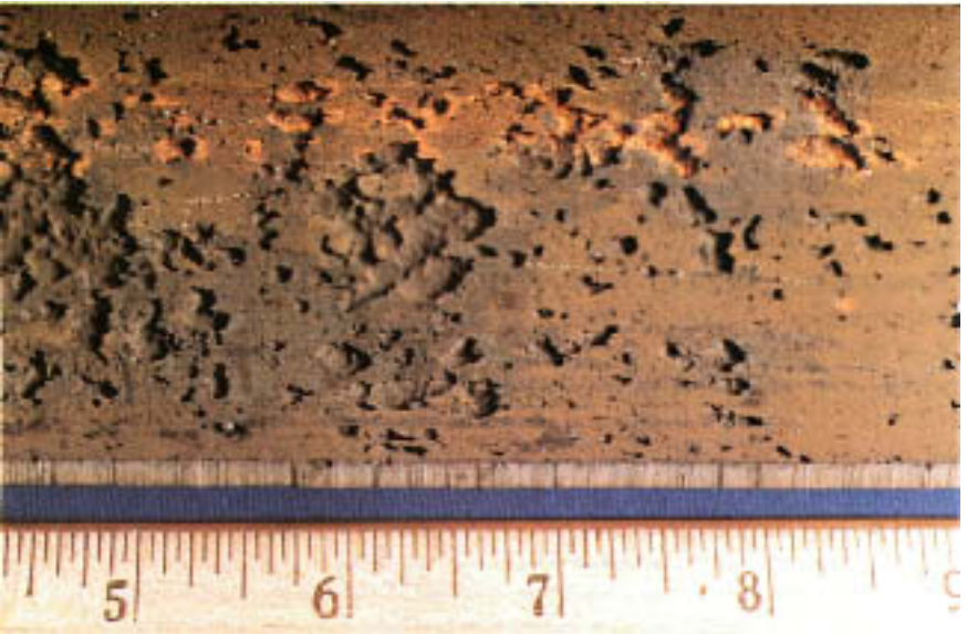
Figure 5.7 Internal surface of downcomer tube showing oxygen-assisted chelant corrosion.
