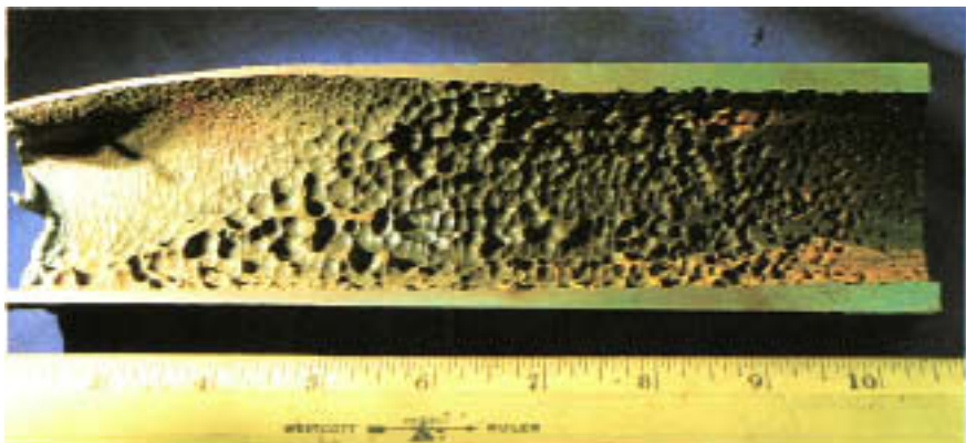
Figure 5.4 Chelant corrosion on internal surface of inlet end.
