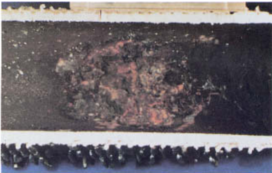
Figure 6.8 Gouging along internal surface opposite fins.
