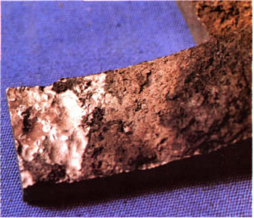
Figure 6.10 Appearance of metal loss on internal surface.
