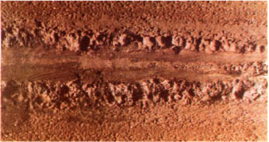
Figure 6.6 Appearance of deposits covering groove.
