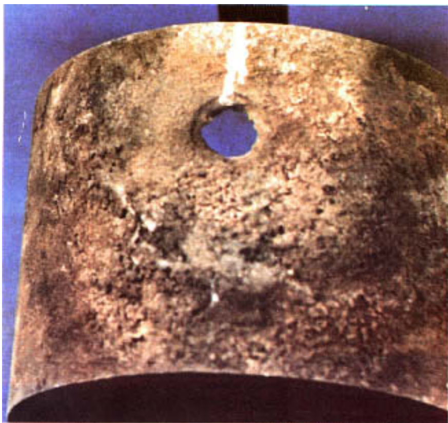
Figure 6.9 Perforation resulting from corrosion of internal surface.
