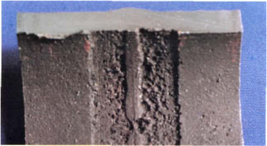
Figure 7.8 Acid corrosion at welds.
