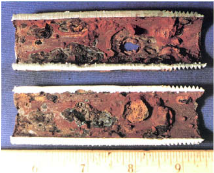
Figure 8.9 Internal surface of condensate line.
