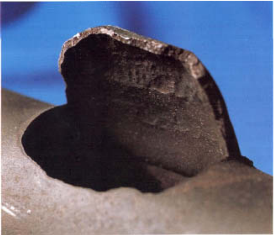
Figure 14.2 Thick-walled burst resulting from hydrogen damage. Note areas of gouging adjacent to burst on internal surface. (Courtesy of Electric Power Research Institute.)
