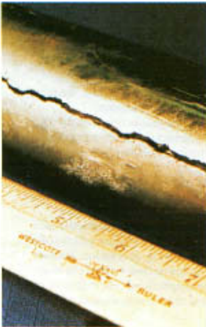
Figure 16.3 Extensive longitudinal crack in a stainless steel soot-blower line. Note that the crack edges have spread apart.
