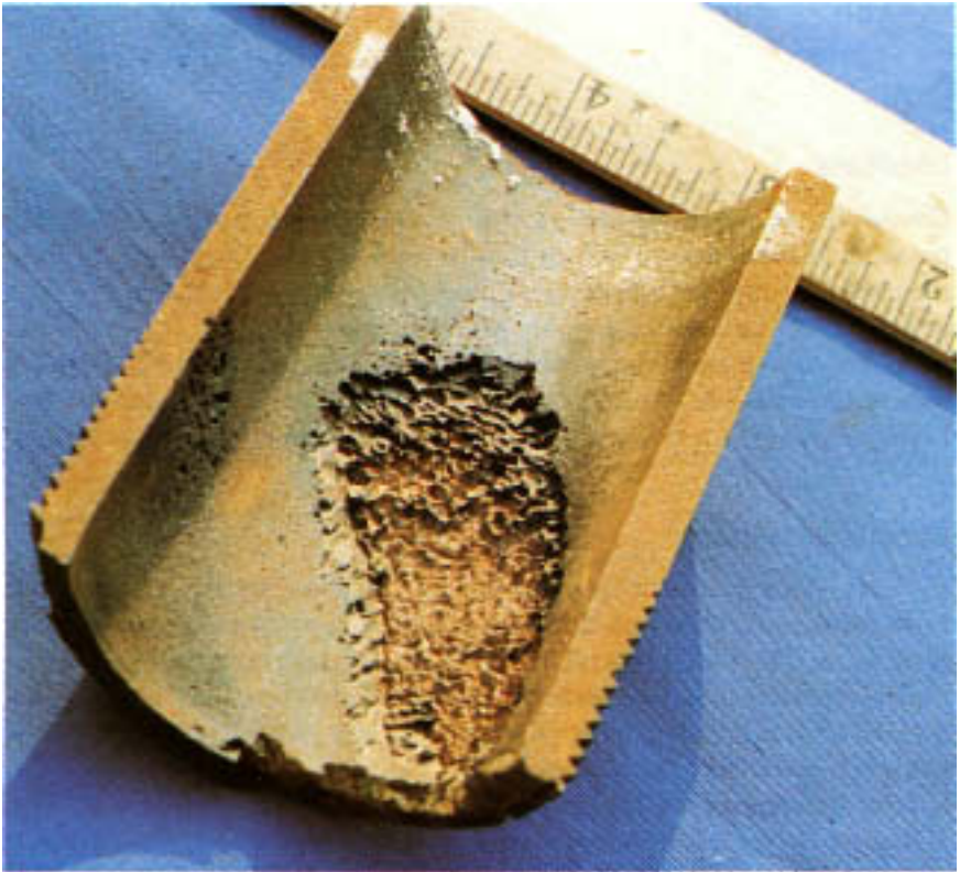
Figure 18.1 Longitudinally split blowdown line with severe localized metal loss caused by cavitation.
