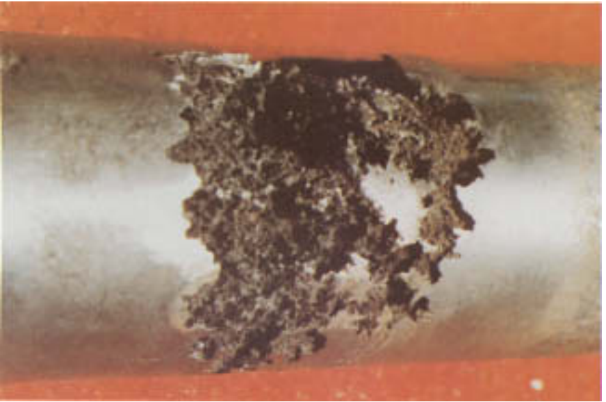
Figure 18.5 Highly localized cavitation damage on steel feedwater-pump shaft. Adjacent regions are free of metal loss.
