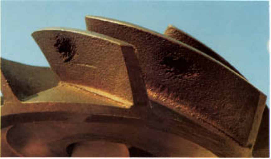
Figure 18.4 Vane damage on low-pressure sides of small, special-purpose, bronze feedwater-pump impeller. Some vanes have been penetrated.
