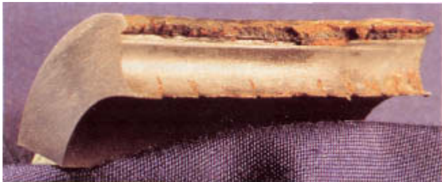
Figure 19.7 Smooth curved contour of defect. (Courtesy of National Association of Corrosion Engineers.)
