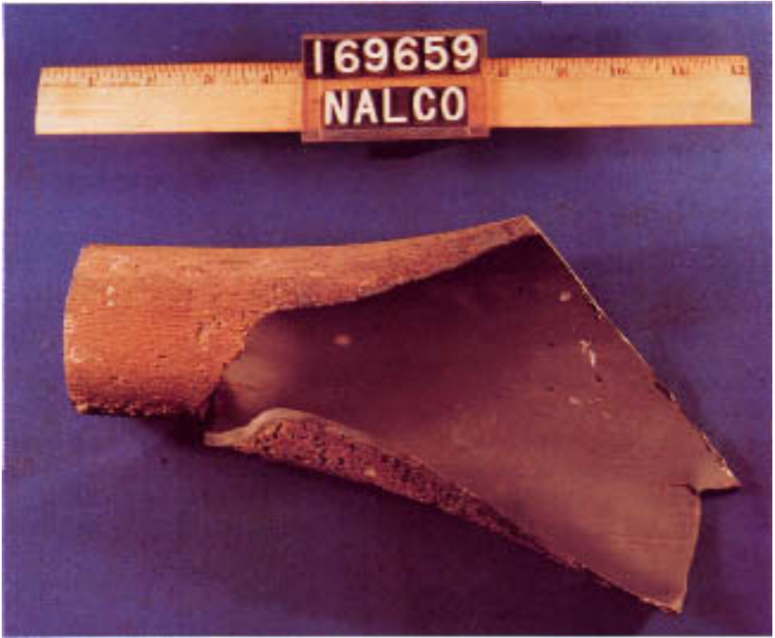
Figure 21.2 Part of a thick-walled rupture in a superheater tube.
