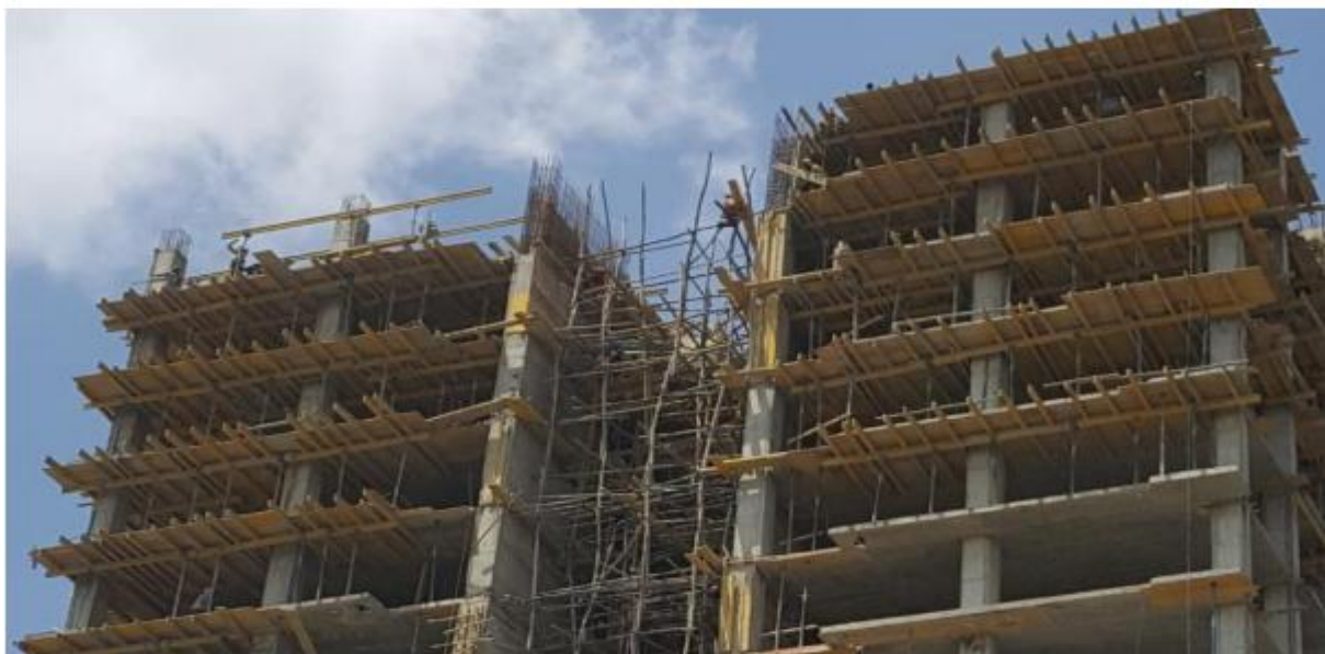
Figure 4.2 formwork materials uses in A.A
