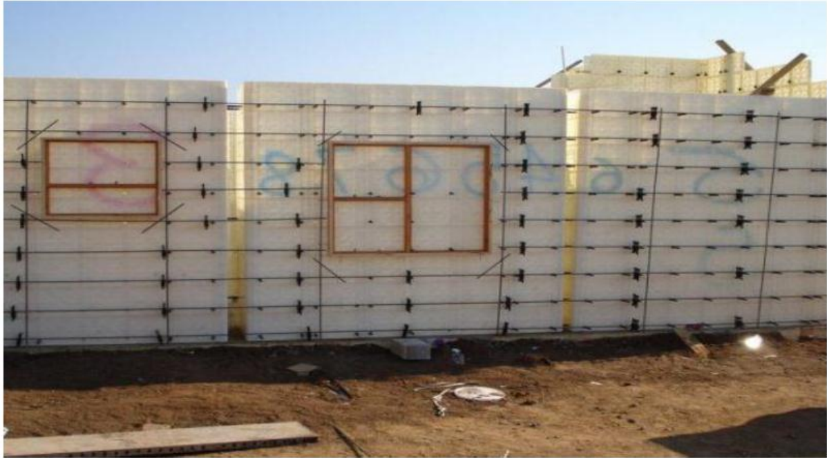
Figure 2.7 Plastic Formwork
