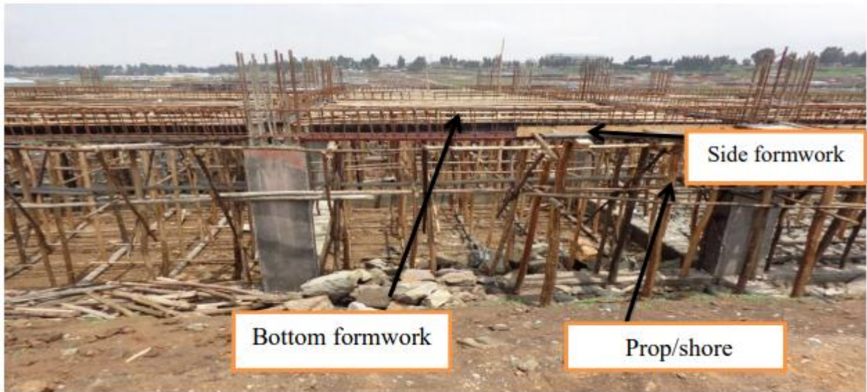
Figure 4.8: Slab and beam formwork bole site.
