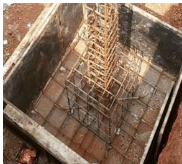
Figure 2.1 Footing pad formwork construction system in Addis Ababa
