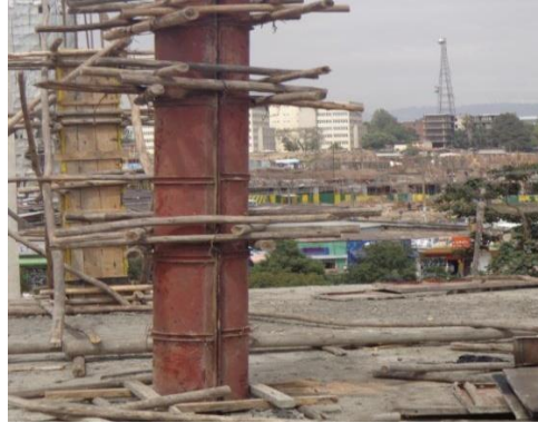
Figure 2.2 Column formwork construction systems in Addis Ababa.
