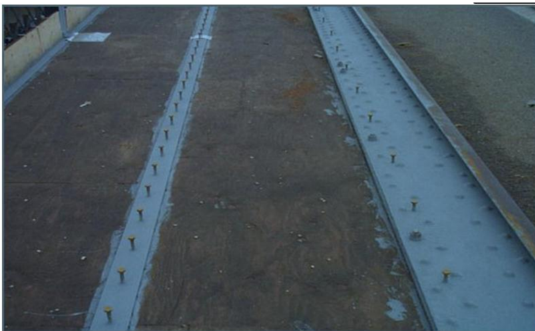
Figure 2.5 Steel Formwork
