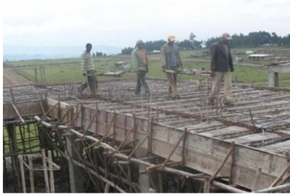
Figure 2.3 Slab formwork construction systems in Addis Ababa
