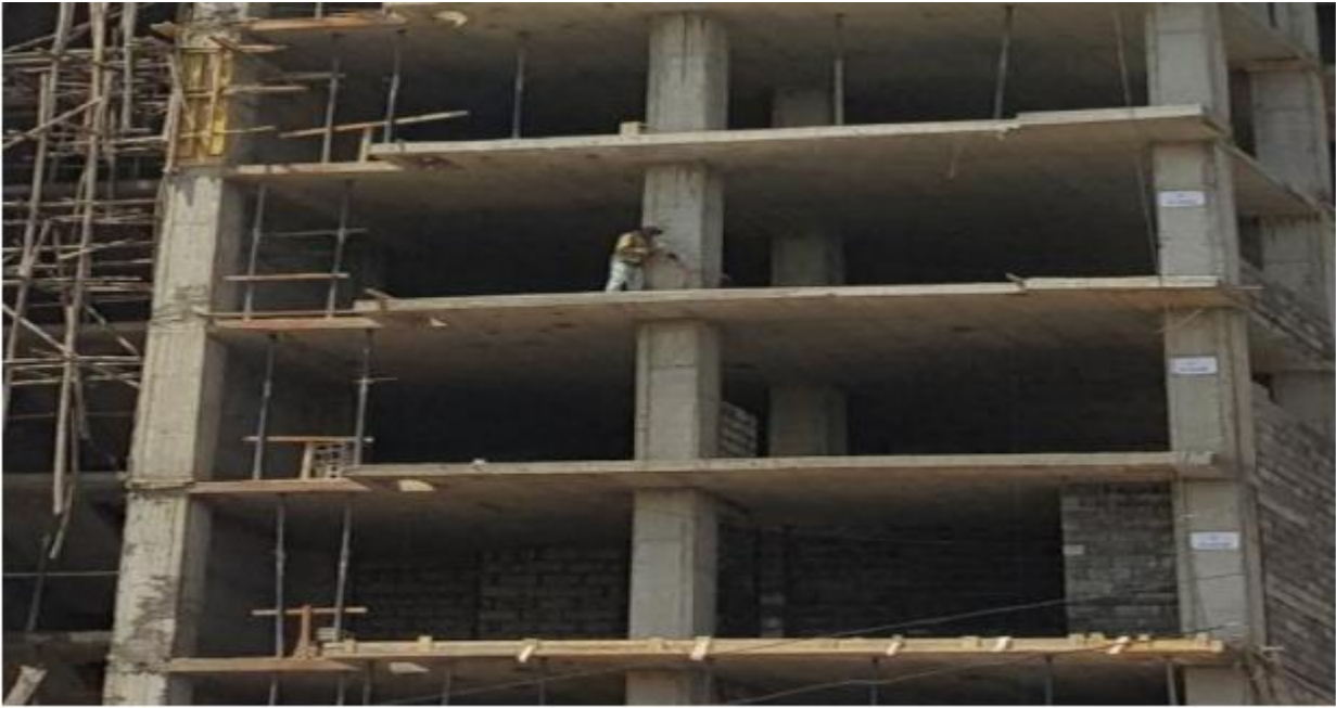
Figure 4.10: Column after stripping of timber formwork at megenagna site
