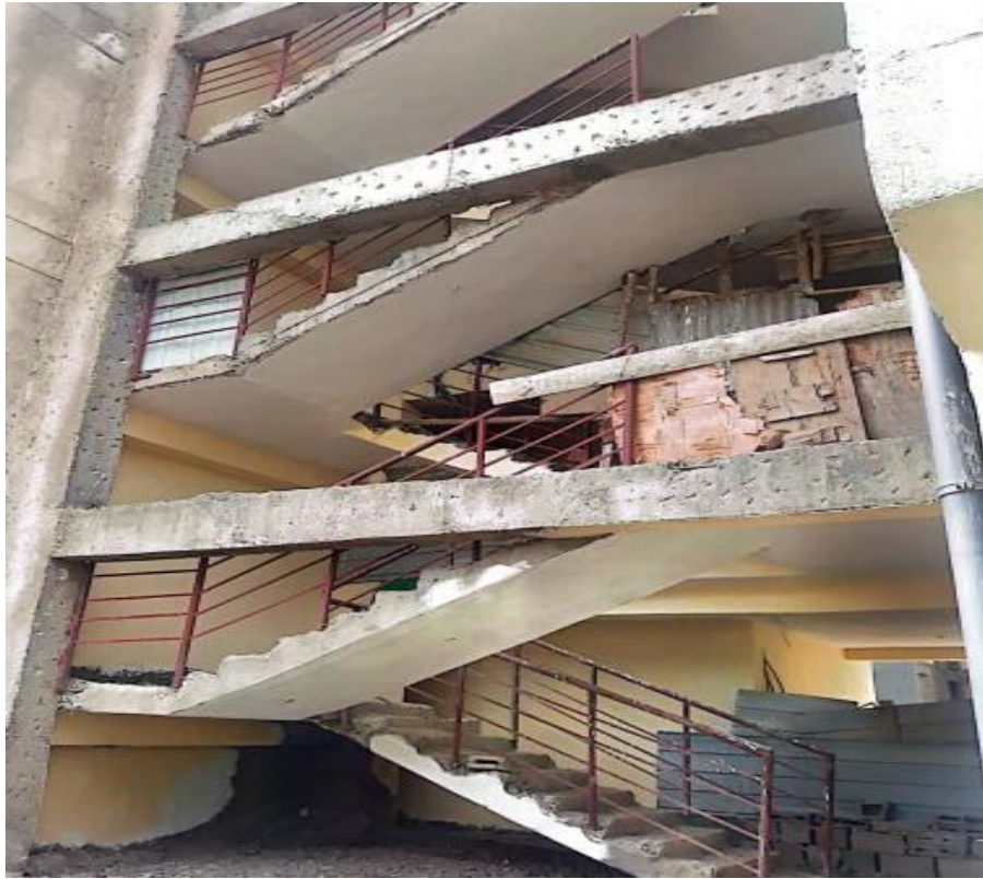
Main Stair case beam
