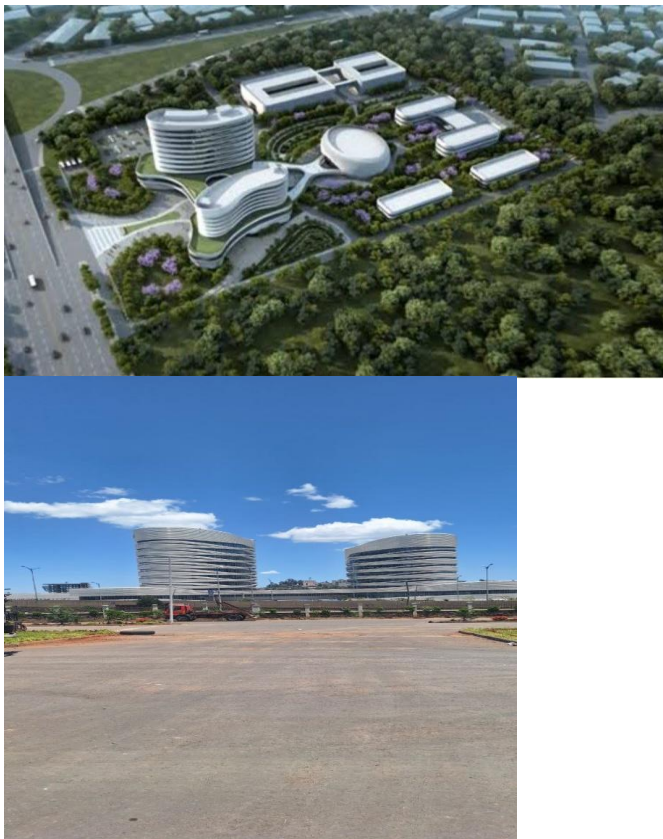
Figure 12: Africa CDC head quarter building
