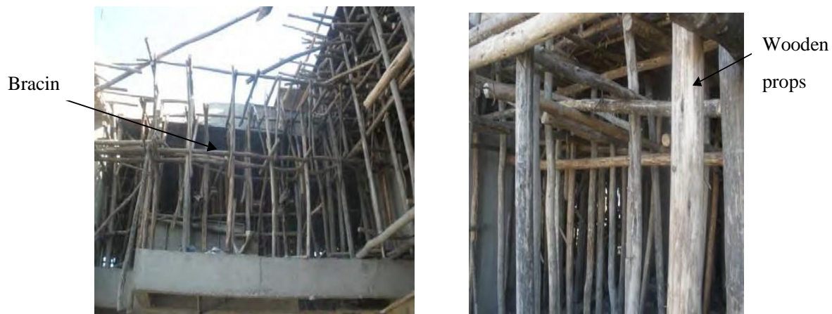
Figure 2. 9 Slab formwork construction systems in Addis Ababa. (Gerji Federal Housing Project)
