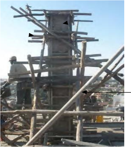
Figure 2. 8 Column formwork construction systems in Addis Ababa (Gerji Federal Housing Project)
