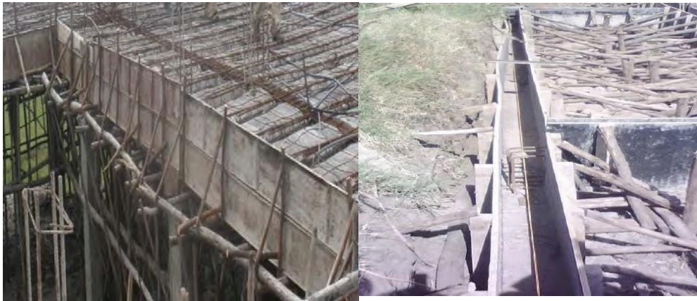
Figure 2. 10 Beam Formwork Construction Systems in Addis Ababa. (Gerji Federal Housing Project)
