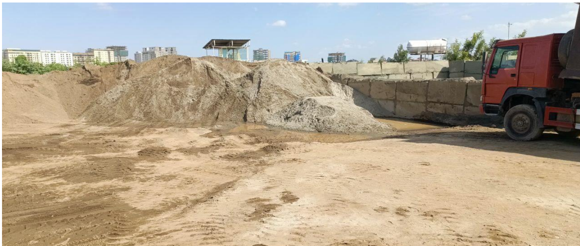
FIG 4.8 sand storage source: prepared by researcher
