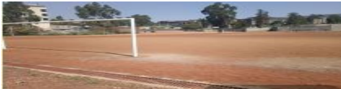
Figure 15 Current Picture of Project Gutomeda sports field, tribune, and fence work
