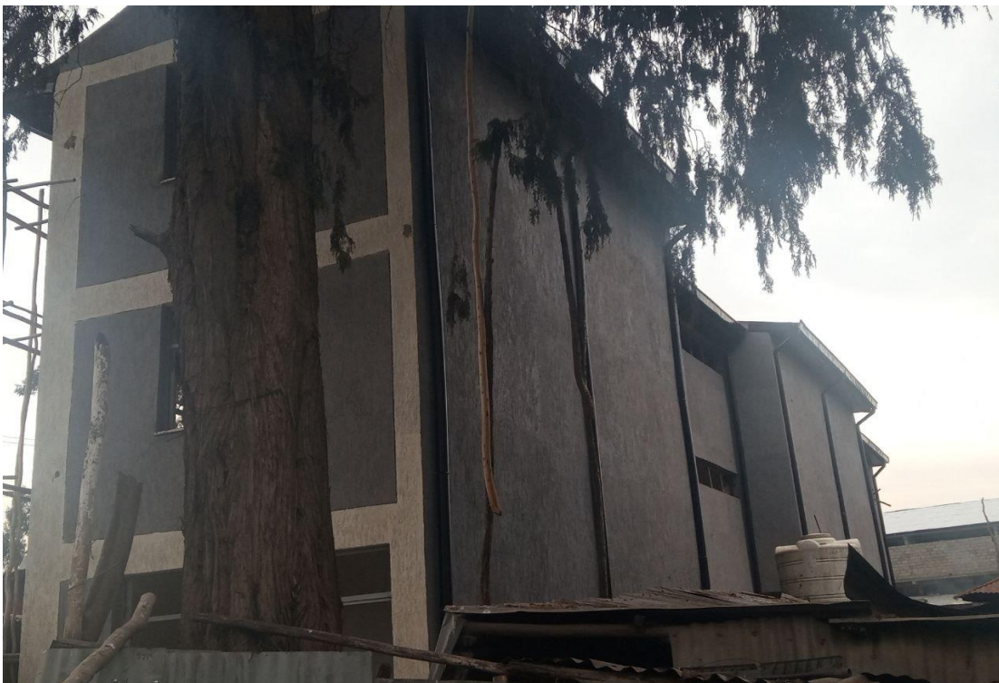
Figure 14 Current Picture of Project pastor police camp G+2 work
