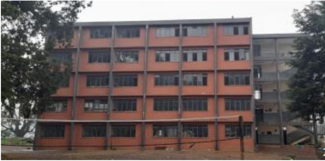
Figure 13 Current Picture of Addis Abeba No 2 School Building Work
