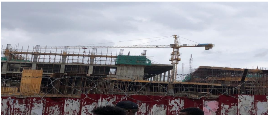
Figure: 4. 8 ADWA ZERO public project under construction
