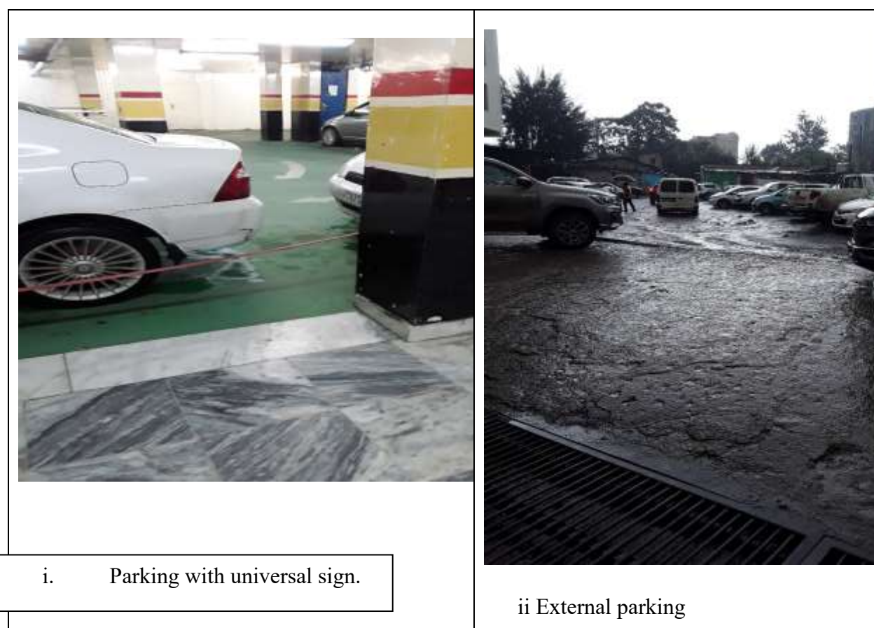
Figure: - 4.23 Sample image for internal and outside the building parking
