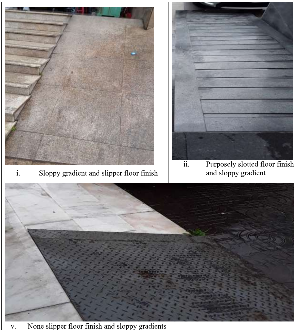
Figure 4.25: - Sample image for ramps observed
