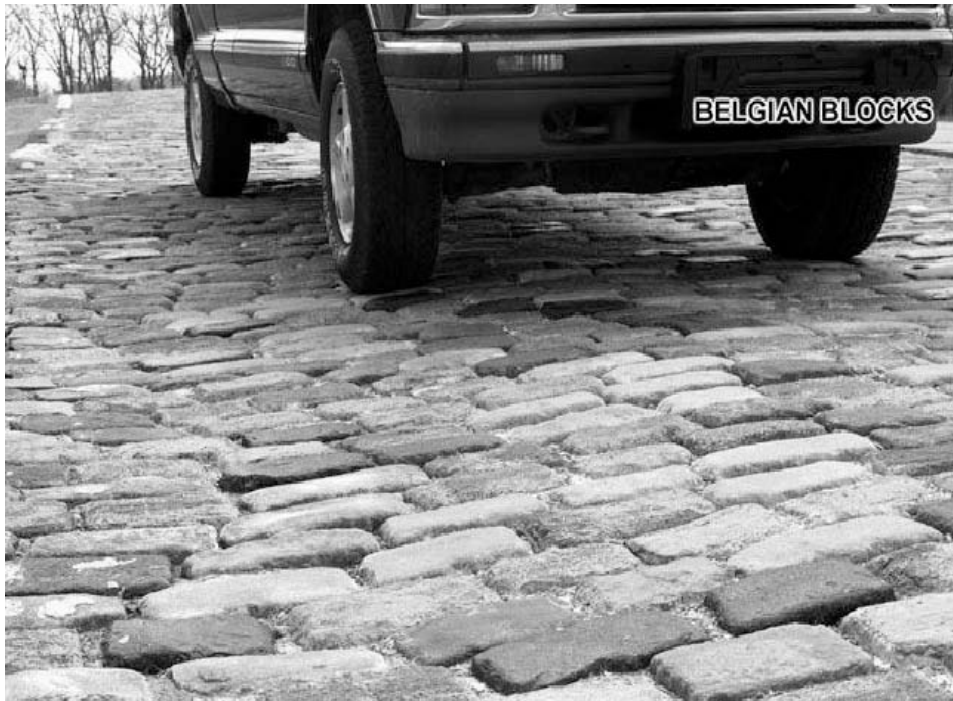
Figure 2.1 Example of fatigue loading event.
