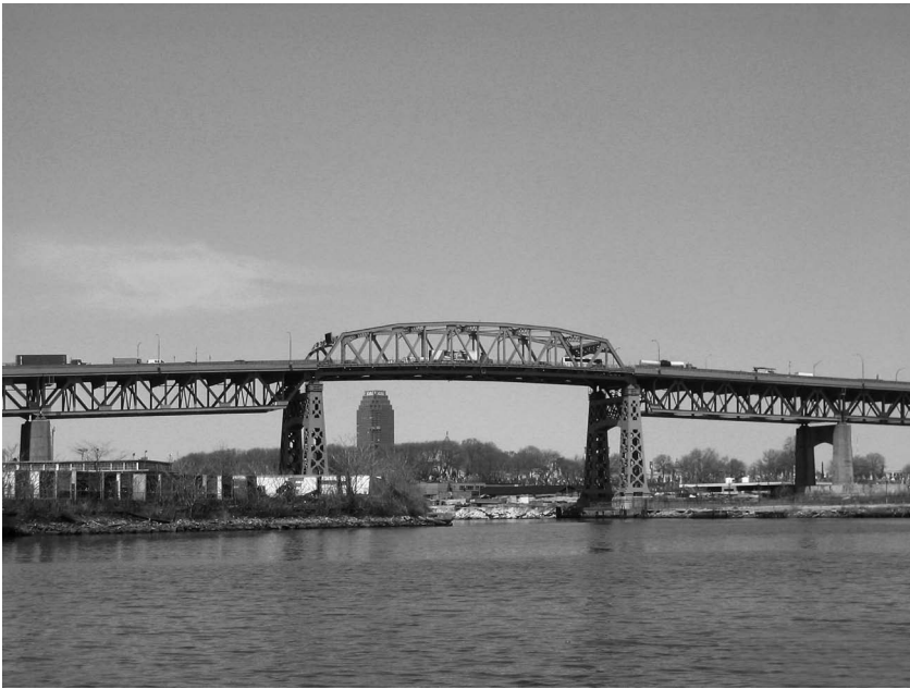
Figure 10.1. Upper: The twin-span Cattaraugus Creek Bridge, carrying Route 219, an expressway in upstate New York. It is pictured in October 2010, just prior to opening, with the old Route 219 bridge in the background. Photo by Frank O'Connor. Lower: A view of the Kosciuszko Bridge on the Brooklyn-Queens Expressway in New York City, taken October 2010. Photo by Steven W. Bennett, PE.
