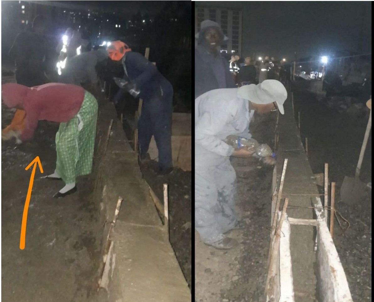
Source: (Bole Arabssa road projects, own survey)
