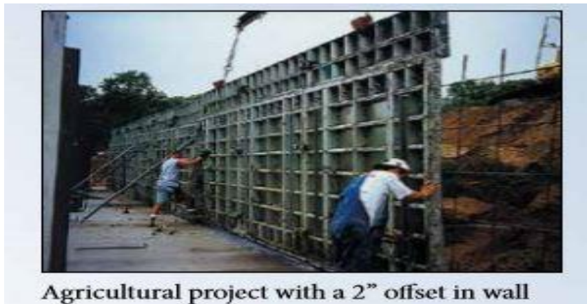
Figure 10. A Aluminum wall formwork parts(Aluminum form work production center)
