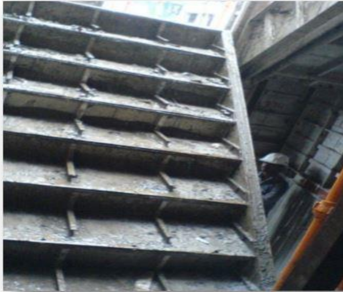
Figure 13. (a) aluminum formwork for staircases
