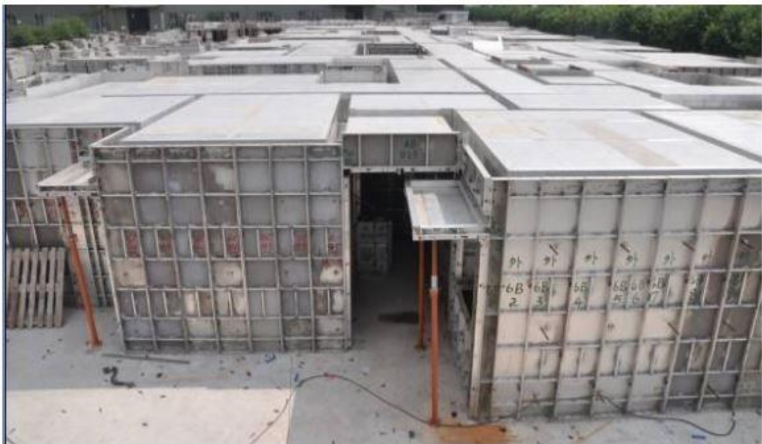
Figure 15. (a) Slab installation (Aluminum form work production center)
