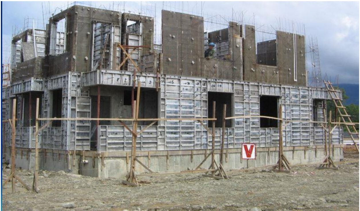
Figure 17. Over all after formwork assembly (Aluminum form work production center)
