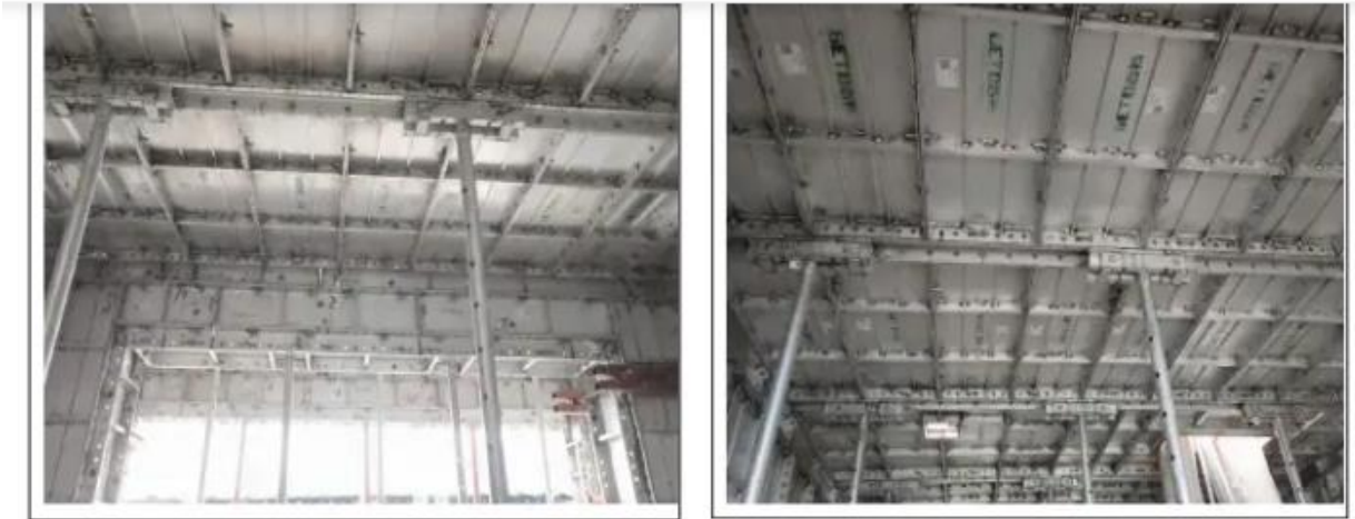
Beam & Slab Assembly
