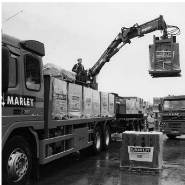
Figure 5.2 Unloading roofing tiles
