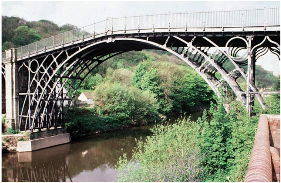
Figure 10.1 Iron Bridge, Shropshire across the River Severn, cast at the nearby Coalbrookdale Works in 1779.
