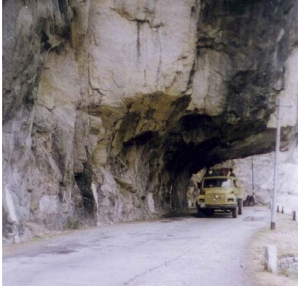
FIGURE 25.1 Photograph of a half-tunnel along hill roads in hard rocks.
