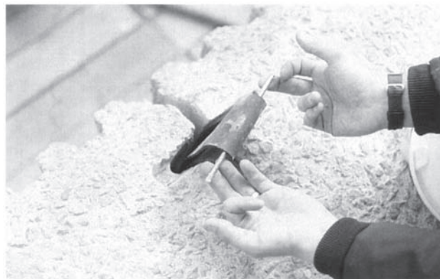
Fig. 1.24 Baffle fixed over stainless steel pin for easy renewal.
