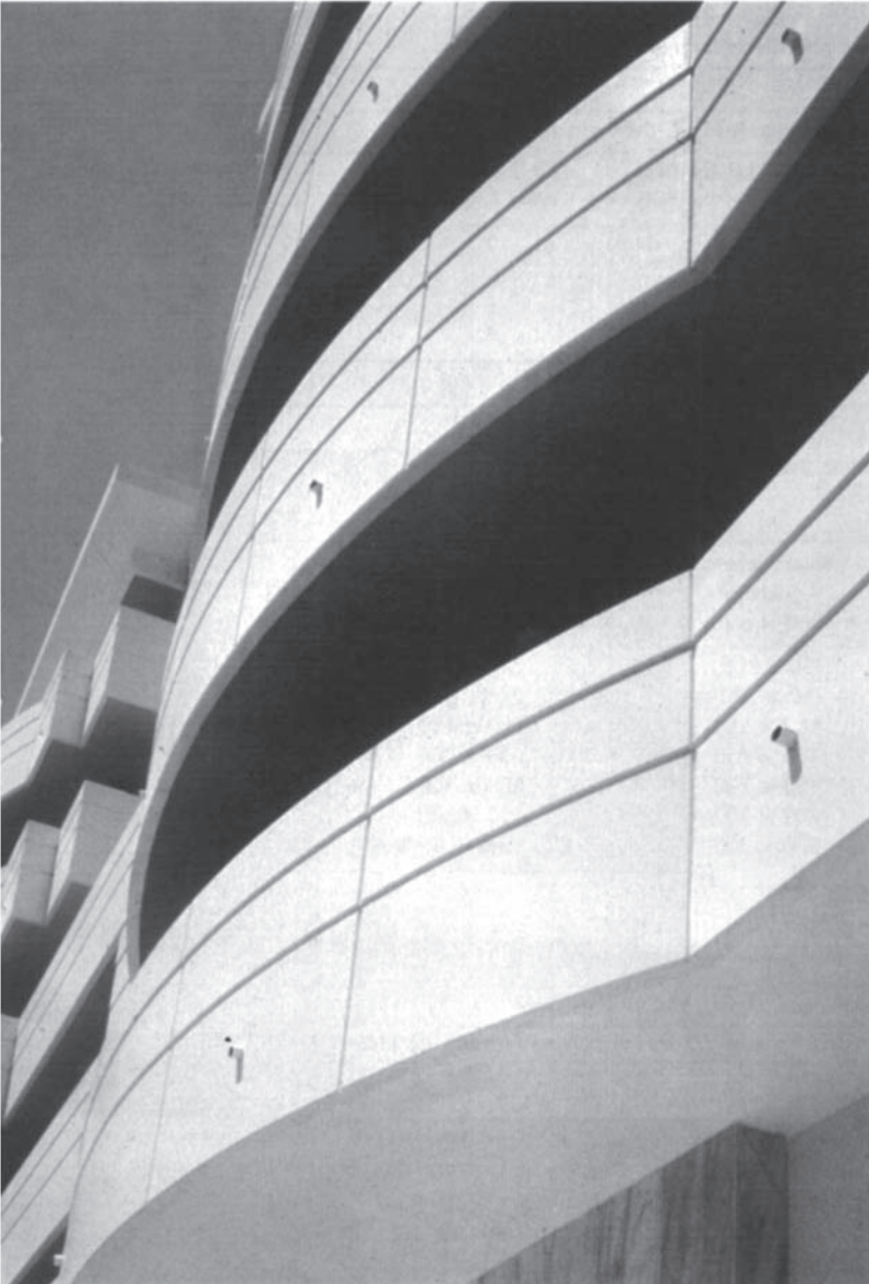
Fig. 3.4 Curved G.R.C. panels..
