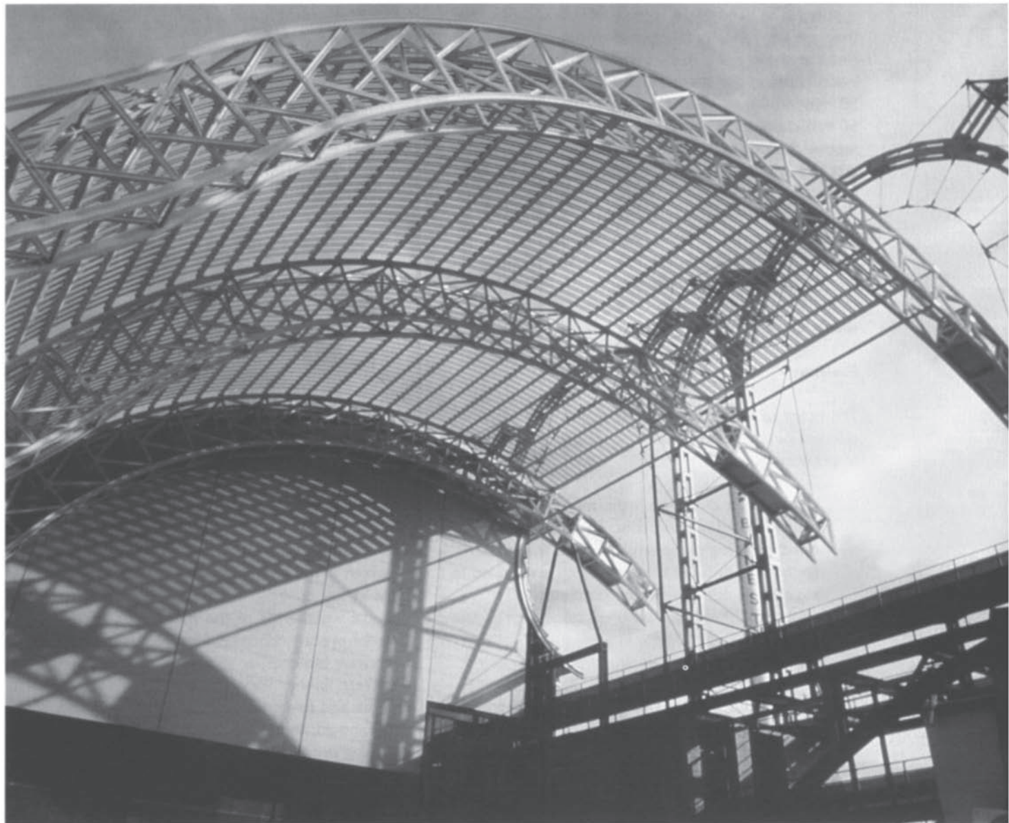
Fig. 1.33 Precast concrete arches at Seville Expo 1992 by Peter Rice.
