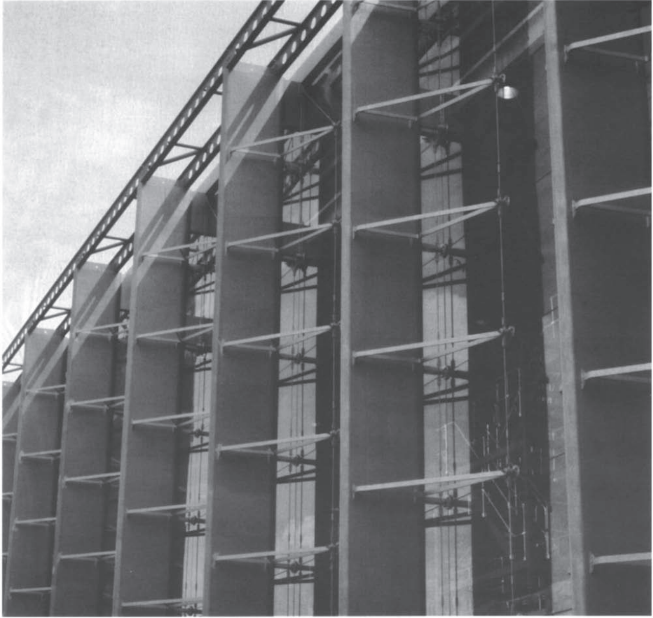
Fig. 6.28a Suspended glazing at Financial Times Building, London (architects: Nicholas Grimshaw & Partners).
