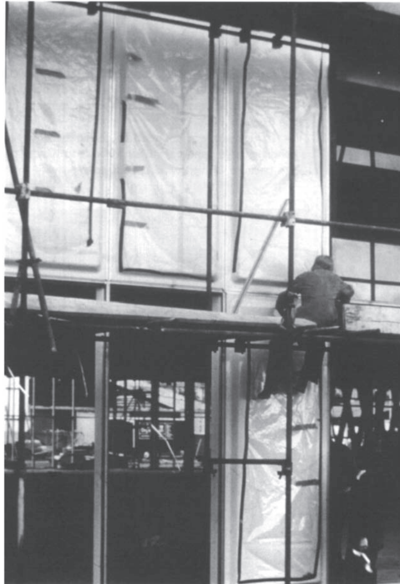
Fig. 2.26 Protection of panels using plastic coating during installation.
