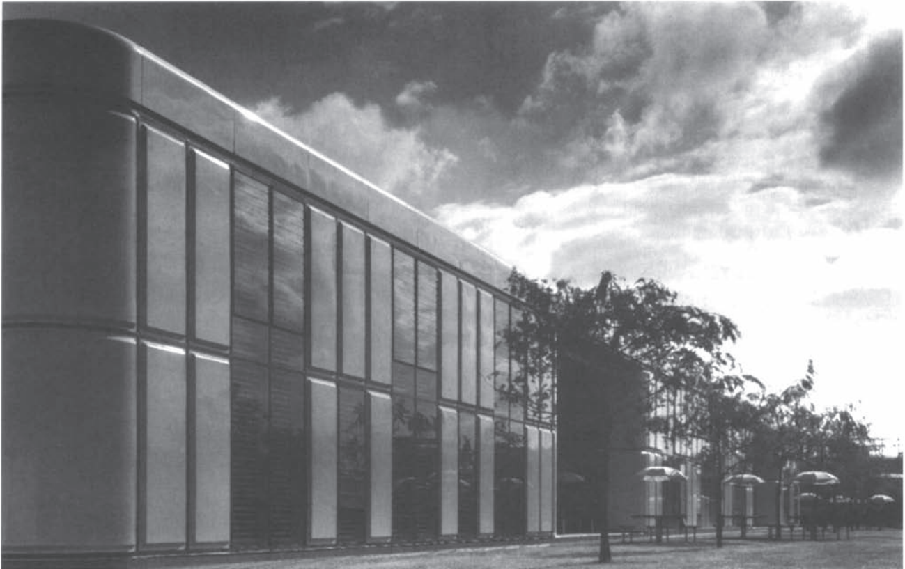
Fig. 2.11 Panels at Herman Miller factory, Bath (architects: Farrell and Grimshaw).
