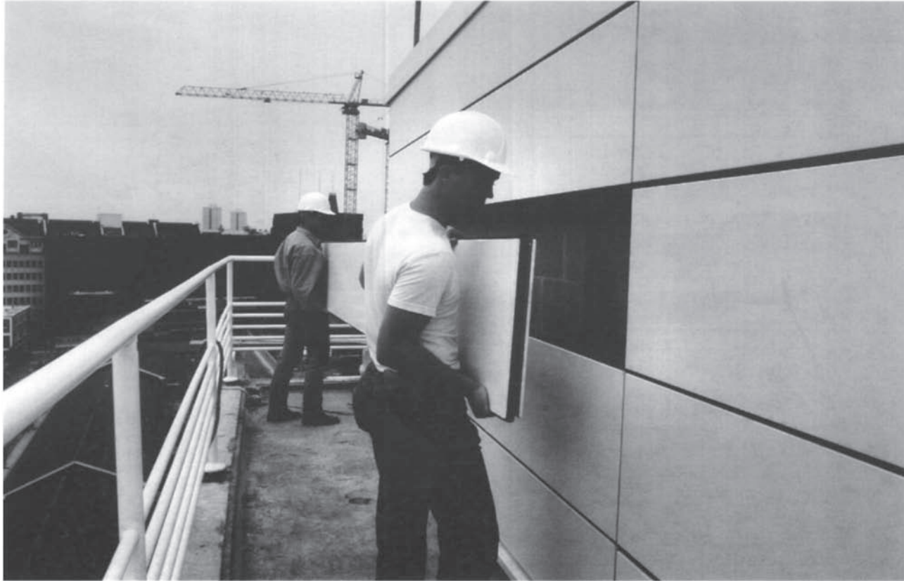
Fig. 5.40 Interchangeable façade panels.
