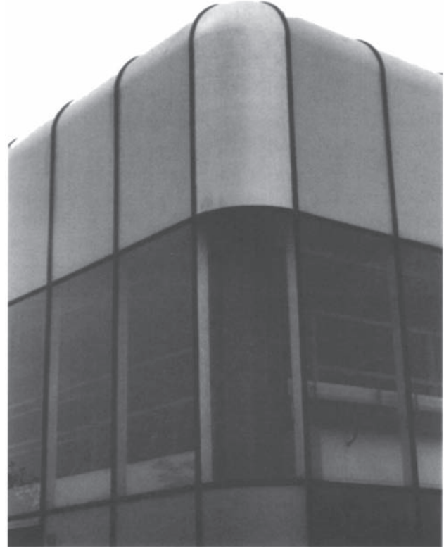
Fig. 2.13 Corner panels at Winwick Quay (architects: Nicholas Grimshaw Partnership).
