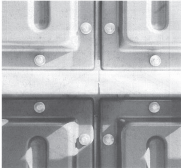
Fig. 4.12 Panels by Superform Aluminium at Financial Times building.
