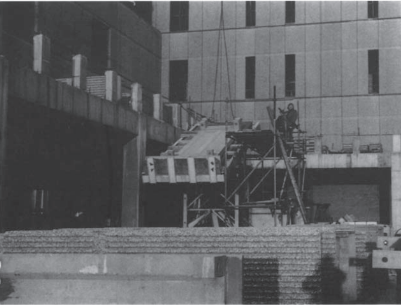
Fig. 1.14 Tilting platform as used at Liverpool Royal Insurance building.
