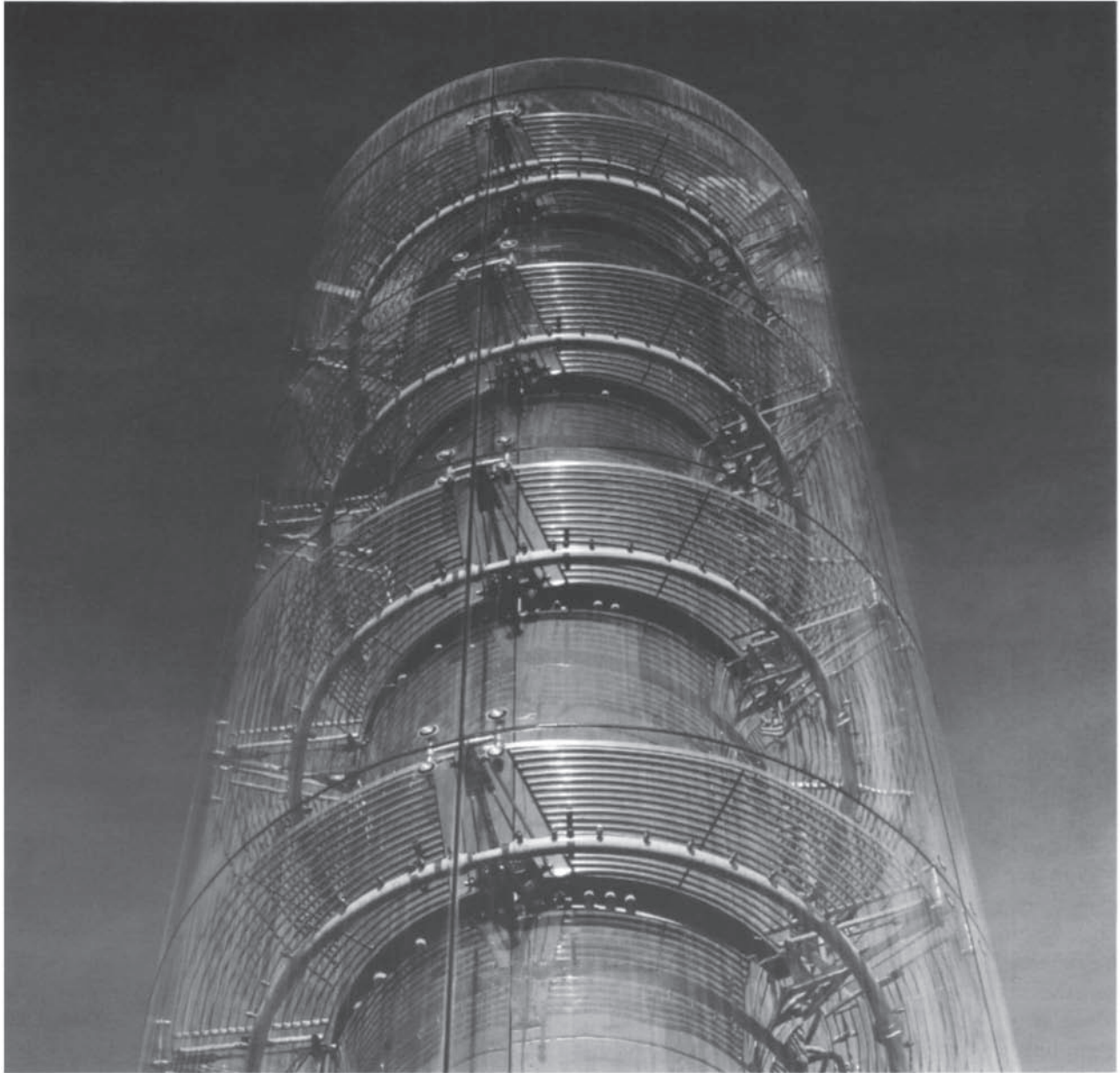
Fig. 6.37 Detail of Thames Water Tower; London (architects: Brookes Stacey Randall Fursdon).
