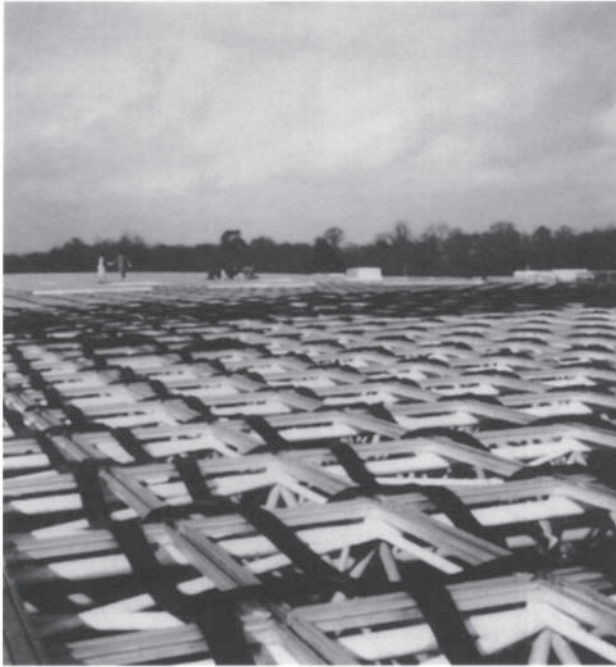
Fig. 5.10 Lattice gaskets used at Sainsbury Centre.
