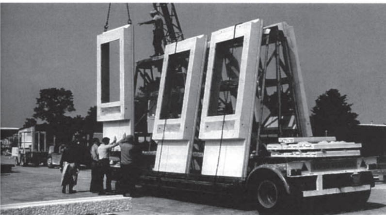
Fig. 1.8 Wall panels being loaded onto A-frame trailer.
