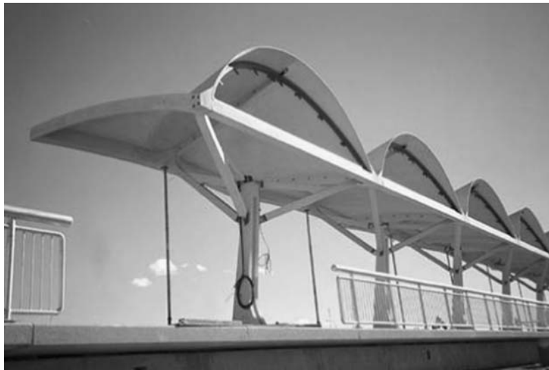
Figure 6-32 The thin-shelled canopies of the Shawnessy Light Rail Train Station in Calgary, Canada
