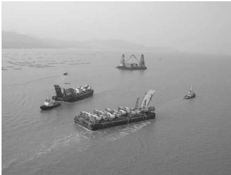
Figure 3-14 Delivery of concrete to an ocean construction site using a ferry (photo provided by Ove Arup, HK)
