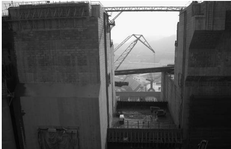
Figure 9-2 Application of new HBC concrete in the Three Gorges Dam
