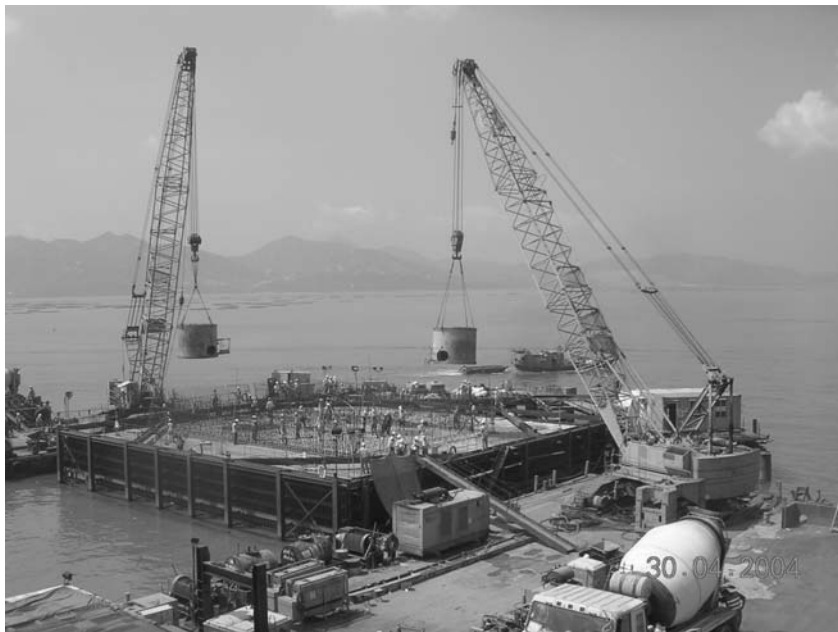
Figure 3-18 Unloading concrete (photo provided by Ove Arup, HK)
