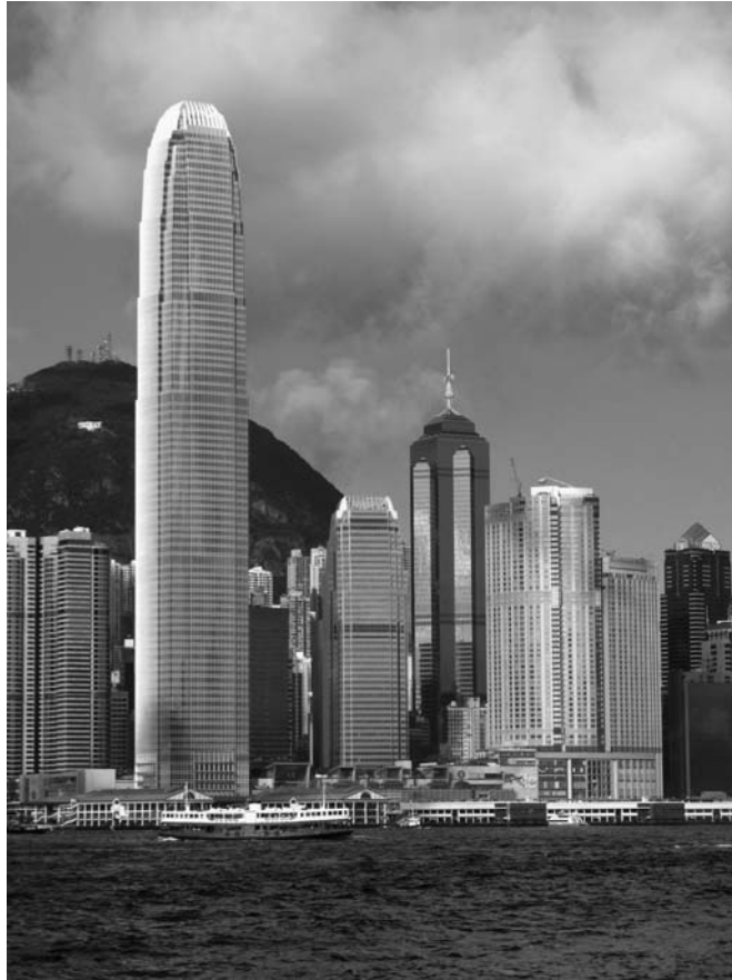
Figure 1-6 International Finance Center, Hong Kong (Photo courtesy of user WiNG on Wikimedia Commons, http://commons.wikimedia.org/wiki/File:HK_ifc_Overview.jpg )
