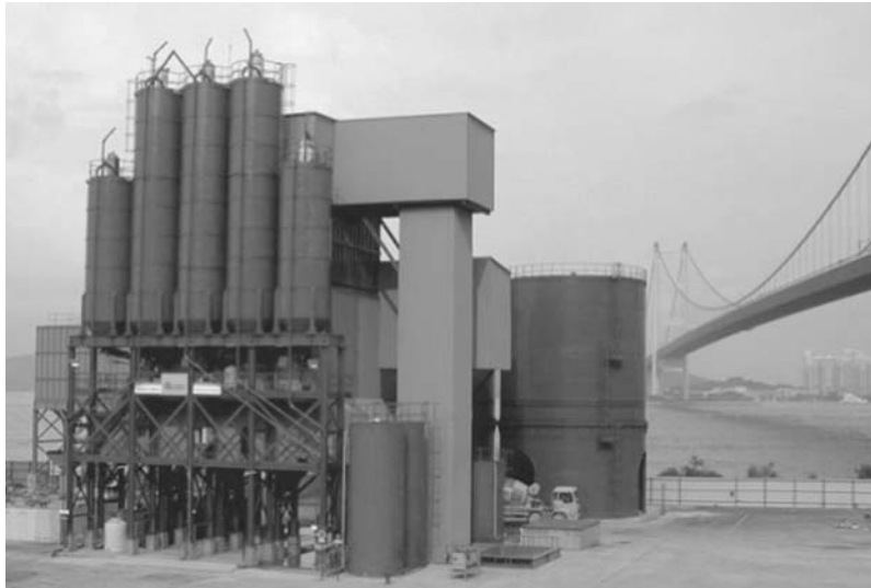
Figure 3-11 Ready-mix concrete plant
