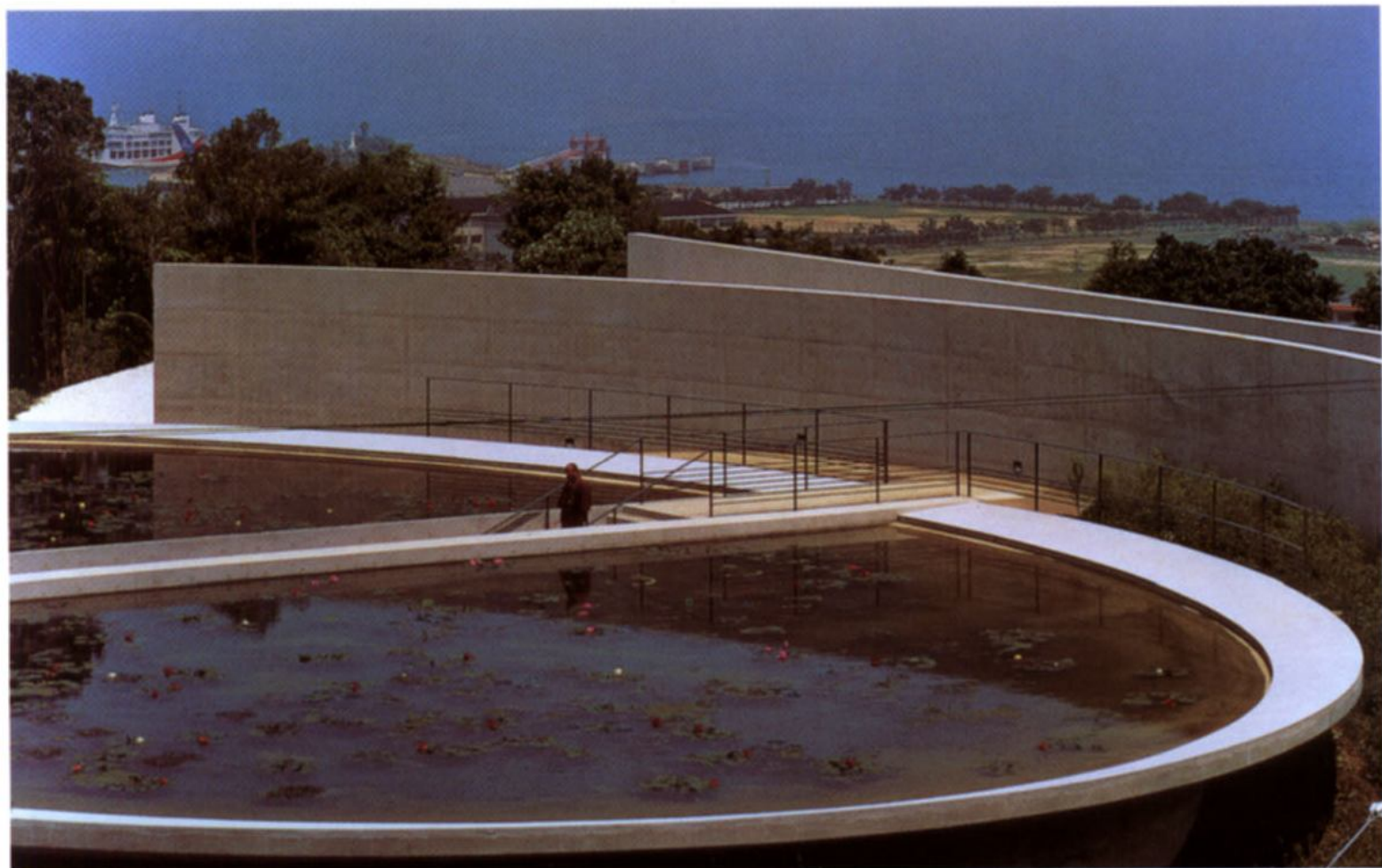
Tadao Ando Hoppuku-ji Temple Awajishima, Japan, 1989–90 The entrance to this temple leads the visitor to the curving concrete wall seen to the left, before he discovers the artificial pond and the stairs, which lead down into the temple itself. There, a representation of Buddha sits, with its back to the setting sun.
